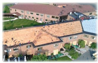
During the first week of June, Christian Care completed a significant roofing project that replaced the entire roof of the main building. This important work was prompted by damage sustained during a hailstorm. Bill's Roofing, a trusted contractor, was selected to lead the project.
